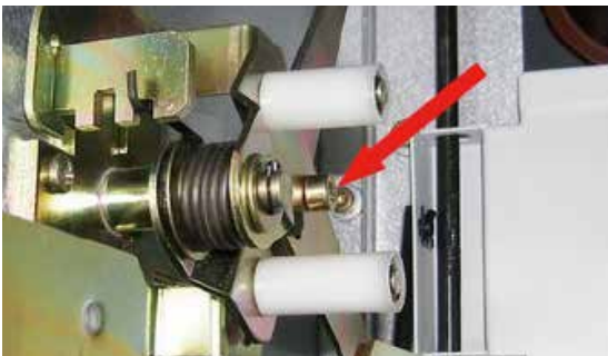
Figure 7.2 : Insert bolts into the overlap holes to disable the shutter mechanism
