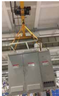
Figure 4.2: Panels Assembly Lifting
