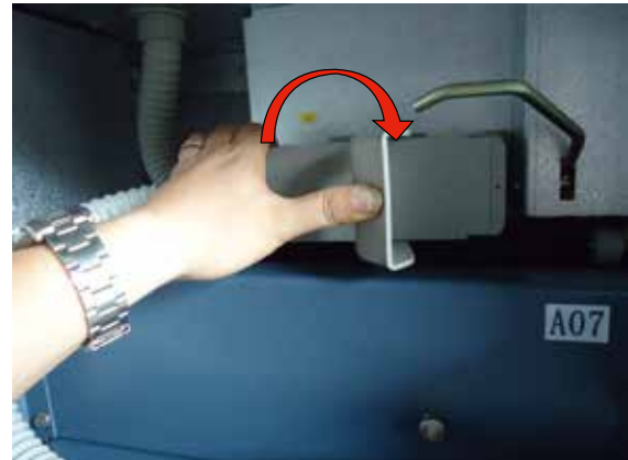
Figure 6.6: Put the secondary plug into switchgear socket
