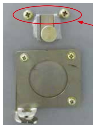
Figure 3.23: Released racking handle Interlock
