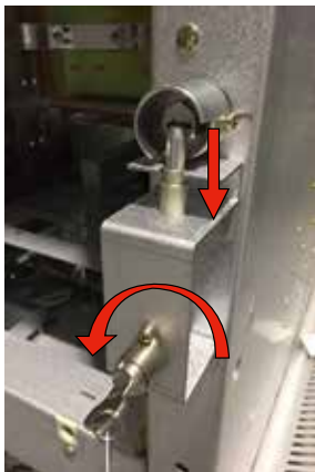
Figure 6.15: Earthing switch closing key lock
