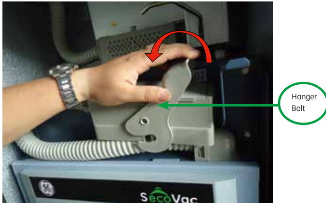
Figure 6.5: Take off secondary plug from truck
