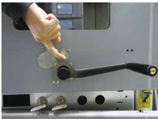
Figure 3.21: Insert the undercarriage handle
