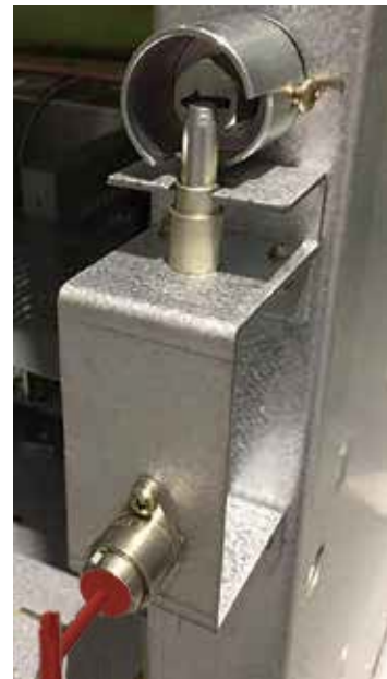
Figure 3.15: Earthing switch closing key lock
