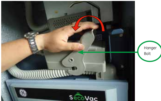
Figure 6.10: Take off secondary plug from truck
